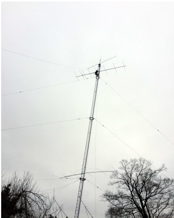
Tram Wire in Place
