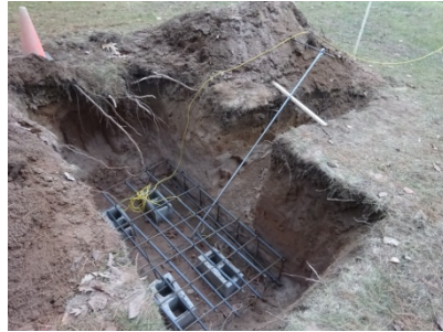
a lot of rebar...
