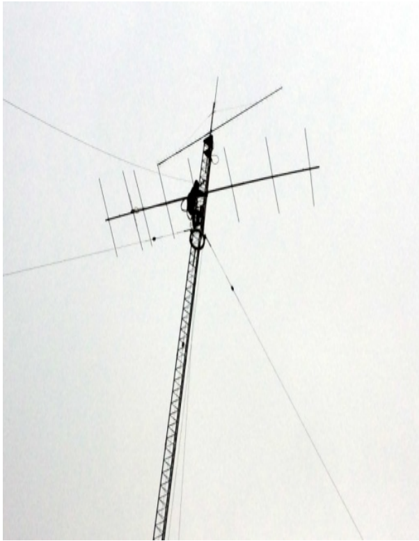
6M Yagi Being Attached
