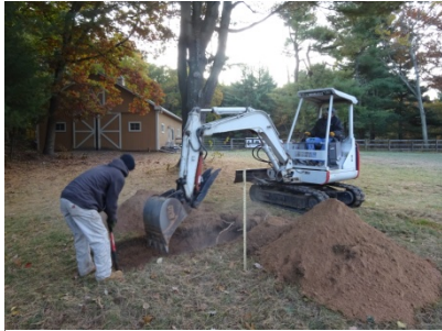
It starts with a lot of digging...
