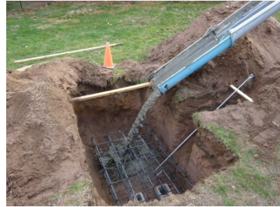
and lots and lots of concrete.
