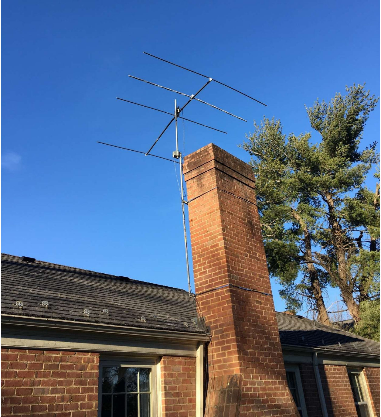
Optional Photo. This could become a Figure 4: The Completed Antenna Following Installation.
