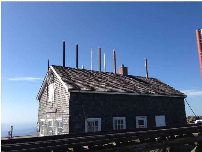
Auto Road Building (radomes sticking out the top) Mt Washington FN44ig
