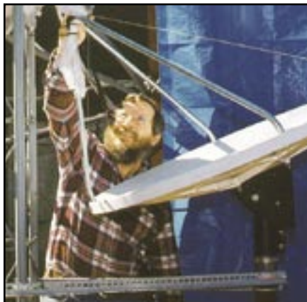
Figure 4 — Offset dish at base of tower under flyswatter (W1GHZ checking focus with string).
