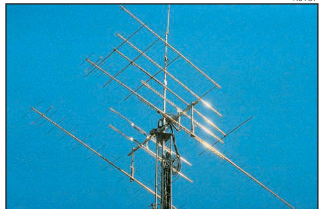
Figure 2—A common rotator loop is the "J" shape as shown here on K3TUF's tower.
